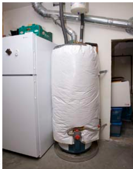
Insulating your hot water tank is inexpensive and easy to do. The money you save will reward your efforts.
